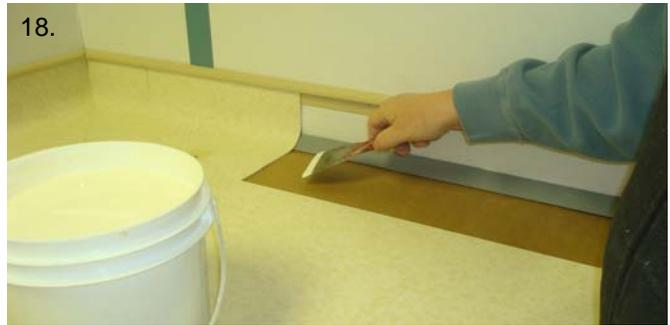
18. Continue to form the tile to complete your run of straight pieces. Let them cool, then apply the correct adhesive to all areas where the flash cove tile is positioned. Continue to tape the pieces together to hold tight seam.
