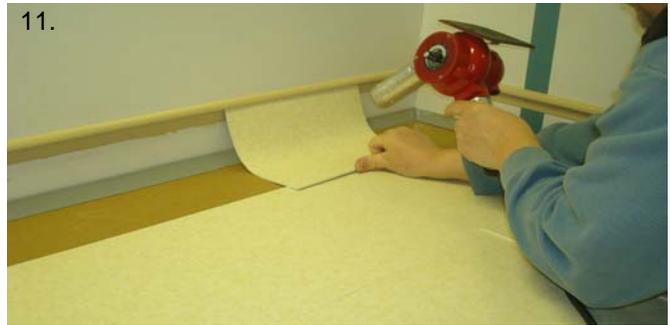
11. Continue to warm the tile until you have the tile in place. Using 1 1/2" masking tape, tape the tile to the installed floor edge as it cools to maintain the shape.
