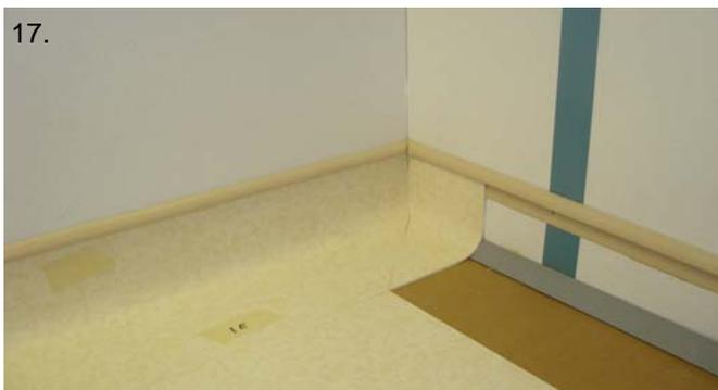
17. Warm up the corner piece bending and adjusting the fit until the tile is in place properly. Tape the seams until the tile is cooled.
