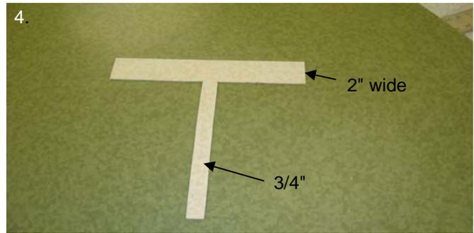
Take one 12 " x 12" tile and create a Tile - T this is used to measure from the top of the cove cap to the edge of the installed tile.
