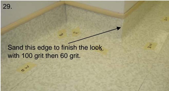
After the detail work is completed use your adhesive and masking tape to hold the pieces in place until the adhesive has set. A small hand trowel or paint brush can work. Be careful not to over glue along seams.
