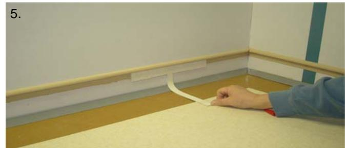
Using your Tile - T push the flat edge under the cove cap following the radius until you meet the tile edge.
