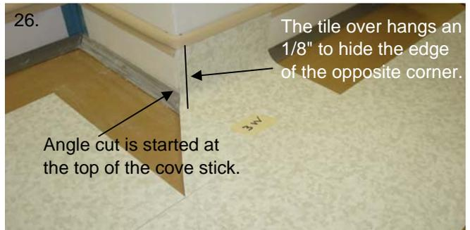
Dry fitting the outside corner pieces and modifications several times is needed for a proper fit.
