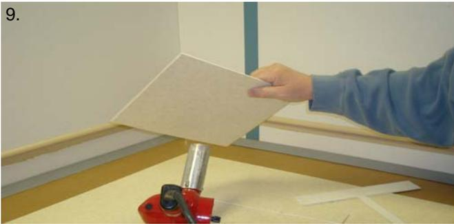
9. With your heat gun warm the tile where the cove stick and the tile will meet until it becomes flexible. Keep the heat moving across the piece.
