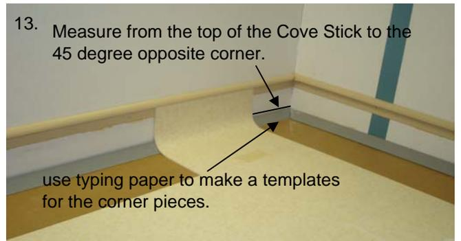
13. Making the first piece for the corner using a piece of paper to follow the contour of the wall.
