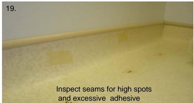
19. Hand roll and inspect any areas for seam movement. Clean and repair adhesive spills or seam blowouts. Follow clean up instructions on the adhesive label.
