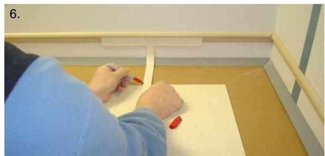
Using your pencil or marking device put a mark on the Tile - T this gives you the total height of the tile that will be formed.
