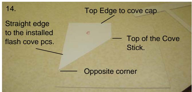
14. Cut out the piece and warm up the piece with a heat gun and install the piece. Adjustments are not uncommon.
