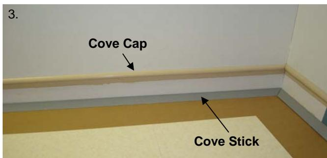
Install Cove Cap and Cove Stick, by using contact adhesive and 1 1/2 " masking tape, staples or brads will work to secure. Let the cove cap and cove stick dry over night.
