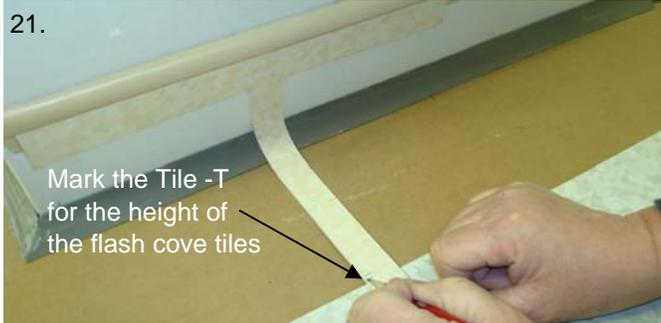
Repeat the same process as above on straight runs by marking the tile-T against the installed tile floor. Tight to the radius. This will influence the high edges during cooling.
