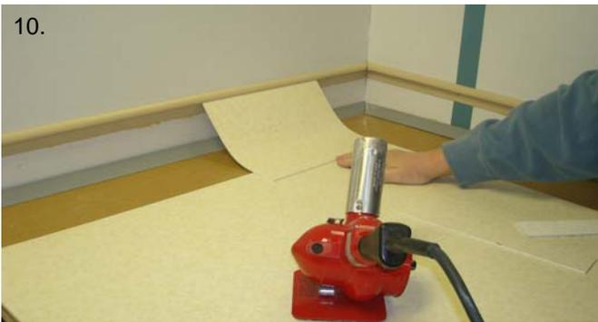
10. Insert the warmed tile under the cove cap and slowly move the tile in place so the bottom edge slides next to and flush to the installed floor.
