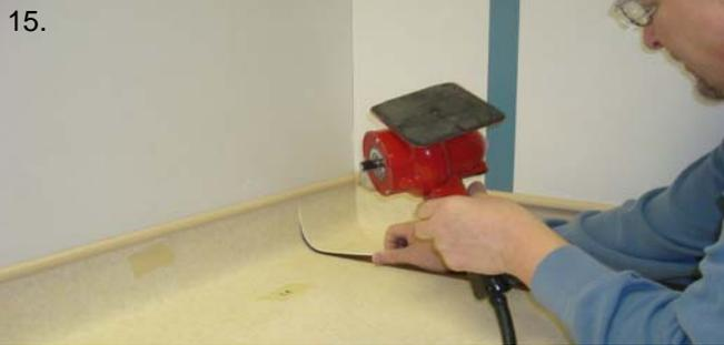
15. Warm your corner piece until it slides into place. Tape to secure and hold the warm corner piece in position until cooled.
