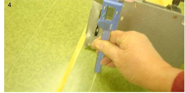
Check the depth of your router cut with a depth gauge and make an adjustment to remove .070 thousands of an inch. Roughly 1/2 the thickness of the tile.
