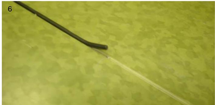
Practice using your floor spatula knife and floor height glide plate for trimming excess material away.
