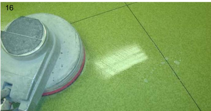
Wet the floor with green prep and conditioner let it sit for 5 - 10 minutes then use a maroon pad and clean the surface using a red pad above the maroon pad for a cushion. The pad will follow the contour of the floor better.
