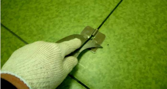
After the weld has cooled, shave off the excess bead with a spatula and height guide. If the bead is shaved before it has cooled, it will shrink below the surface of the flooring. Keep the spatula sharp by periodic honing with a fine sharpening stone.
