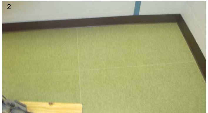
Lay out the field so that the last section ends at least half the length of the tile from the wall to allow space for the use of a router and hot air welding tool around the room perimeter. Tiles can be purchased pre-grooved in 24" or 36" sizes and custom sizes too.
