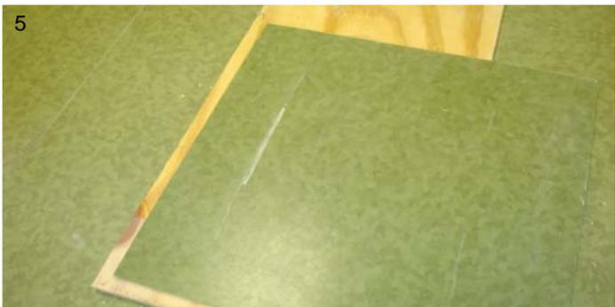
Create a seam weld sample to experiment on achieving the optimum melt flow for your floor conditions
