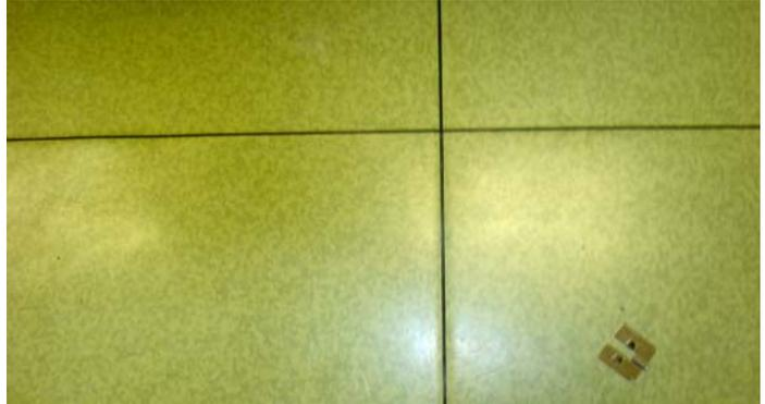
After welding and trimming all the seams in one direction, repeat the router procedure, welding, and trimming procedures on all seams running in the opposite direction.
