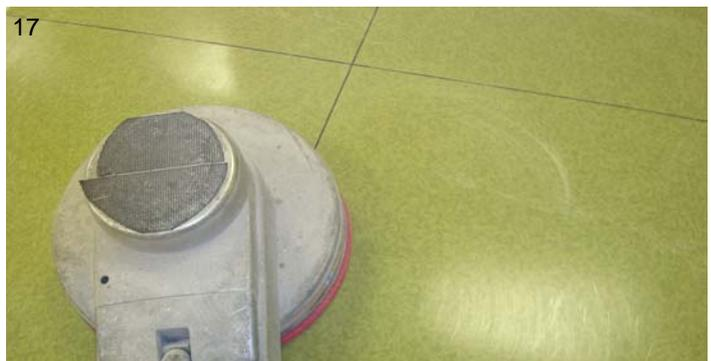
Run 3-4 passes back and forth with the maroon pad, then clean with clean clear water to remove the dirt and film from the floor. Let the floor dry.
