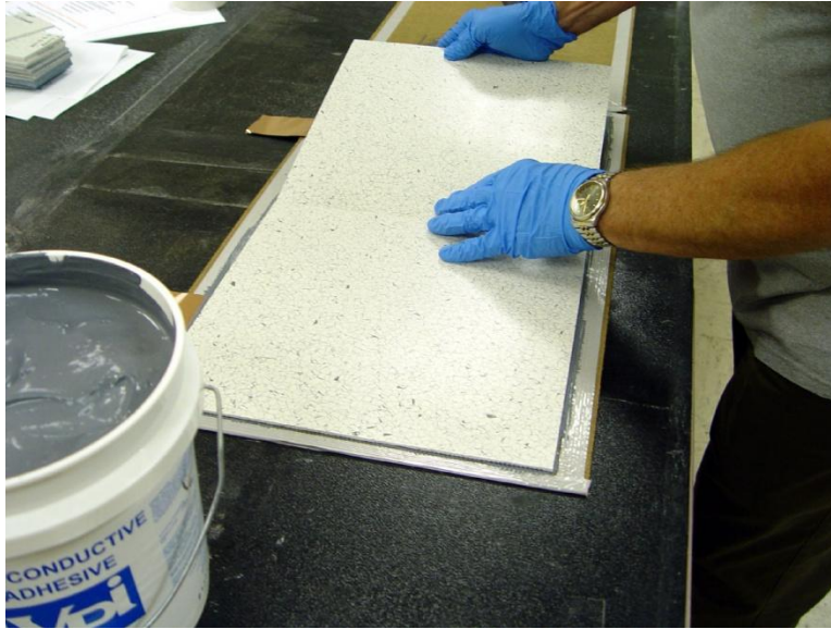
Figure III. Tile Installation
